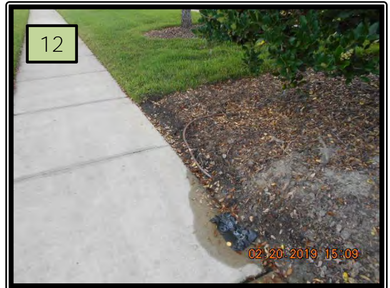
12. Reference Pic (12) Broken irrigation was found in the landscape beds at the amenities center.
