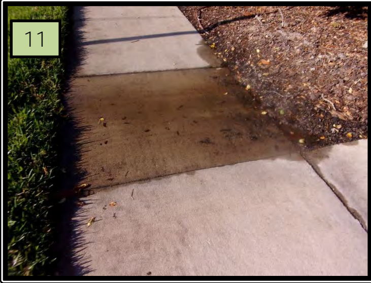
11. Reference Pic (11) Located at the amenities center there is a irrigation repair that needs to be addressed as the water is leaking onto sidewalk.
